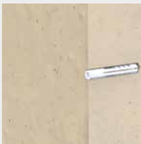
1. Insert suitable dowel
